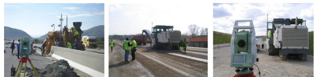
Figure 3. Example of construction of connection roads with 3D-leveling systems
