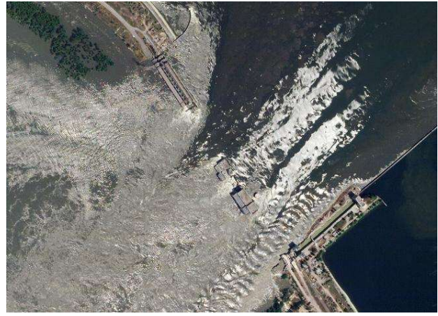
Fig. 2. Destruction of the Kakhovka hydroelectric dam (June 6, 2023)
